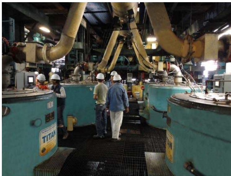
San Cristobal Mill “A” continuous centrifuges
